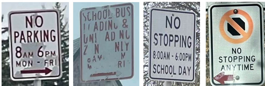
FIGURE 13: SUBSTANDARD PARKING, STOPPING, LOADING SIGNS
