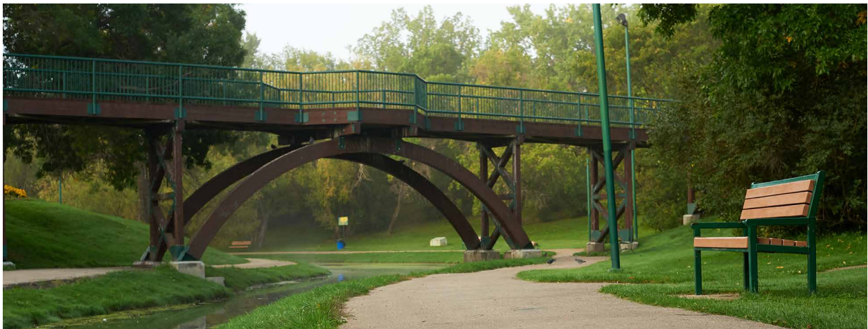
Figure 15: Bridge at Crescent Park.
