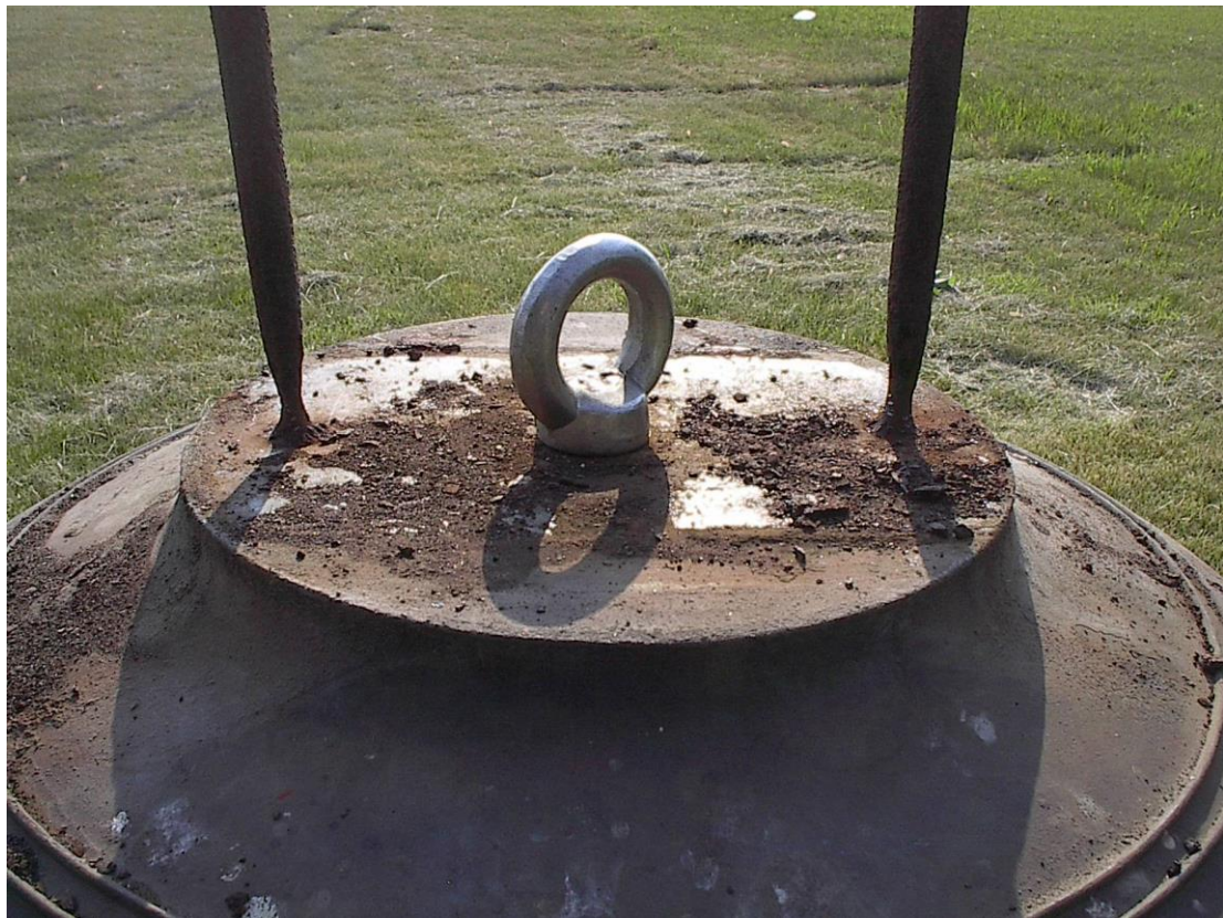
Example of Badly Corroded Bell Support Bolts
