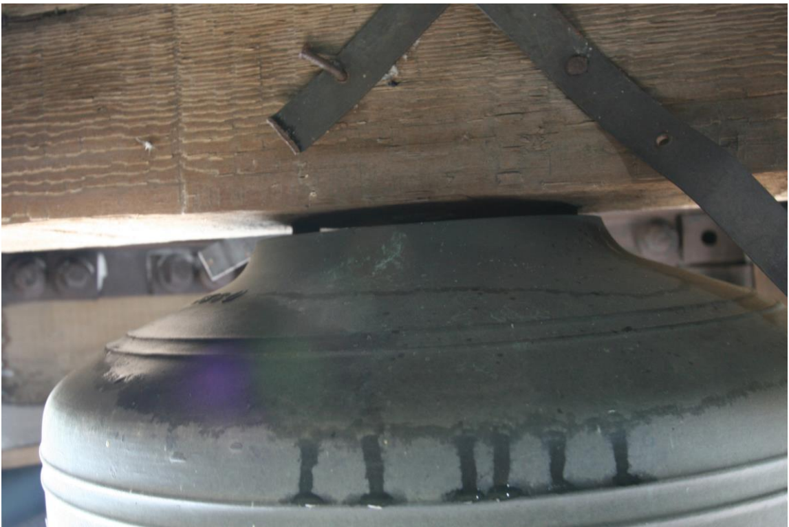
Top of Bell – Space between bell & beam
