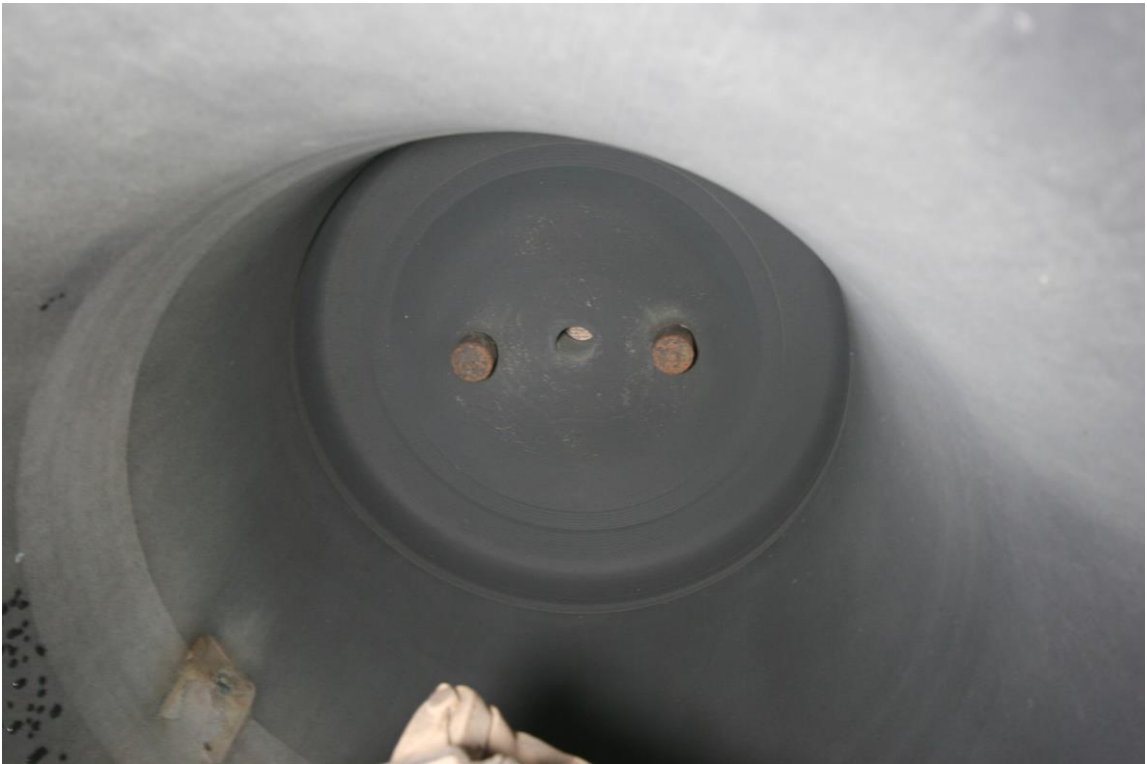
Inside of Bell – Support Bolts
